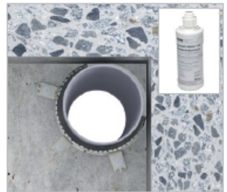
Non-combustible pipes with Wrap into the wall
