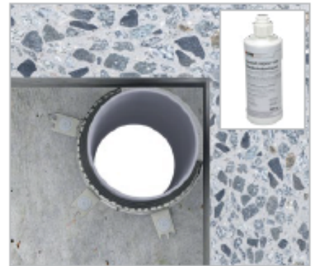
Non-combustible pipes with Wrap into the wall
