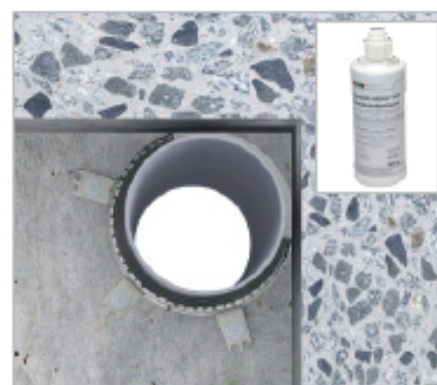
Non-combustible pipes with Wrap into the wall
